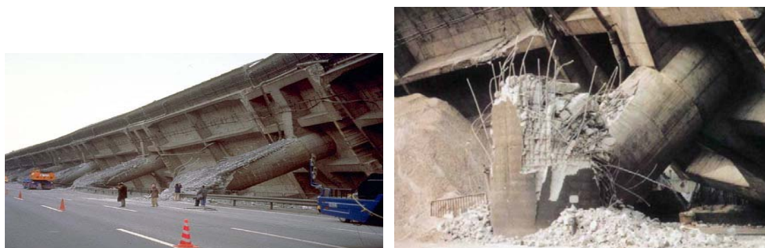
Figure 2.9: Complete Collapse of Bridge, 1995 Kobe Earthquake [CALTRANS, 2006]
